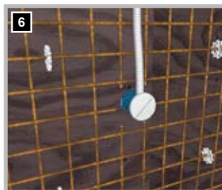
6 Insert the pipes and use as electrical socket or large clamping socket.
