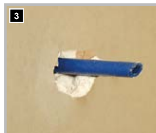
3 The drywall builder makes a hole with a hammer allowing the spike to go through, serving as a center for the drill bit.
