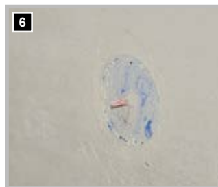
6 The socket is quick to locate using the plaster tongue.
