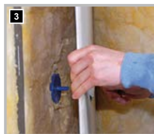
3 The hole for the socket can now be drilled without re-measuring the installation position.
