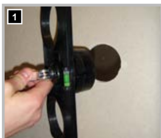
1 Drilling the middle hole
