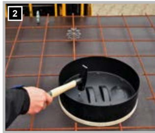
For in situ concrete, nail on to the formwork; for prefabrication plants, glue to the formwork table.
