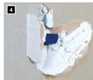
4 The protruding spike serves as a centering for the Ø 68 mm drill bit.
