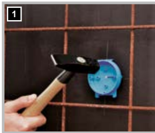
1 Attach device cover to the formwork with nails
