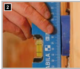
2 ... so that it protrudes approx. 1 cm outside of the masonry.
