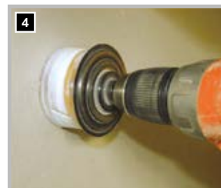
4 You can drill the hole without re-measuring the installation position.
