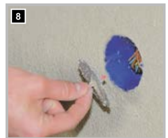
8 ... And remove the plaster film – finished!
