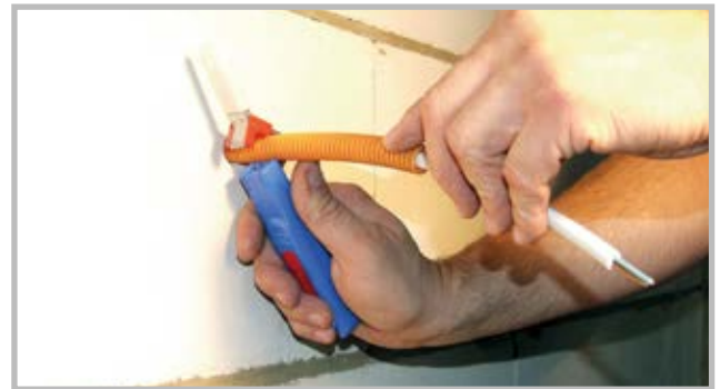
2. Cut the installation pipe flush to the wall.
