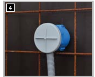
4 Wall installation as electrical socket.
