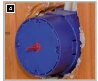
4 The cover will still be protruding approx. 2.5–3 cm.
