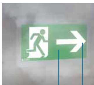
GuideLED \geq 100 \text{ cd/m}^2 \geq 500 \text{ cd/m}^2
