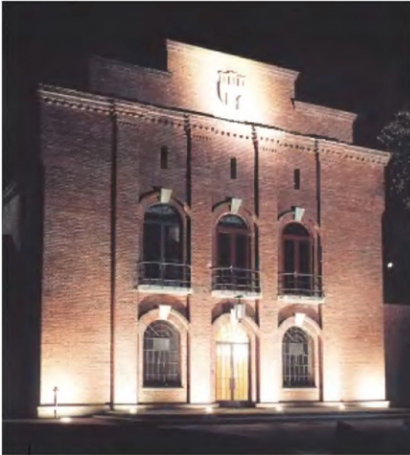
ground recessed luminaire building
